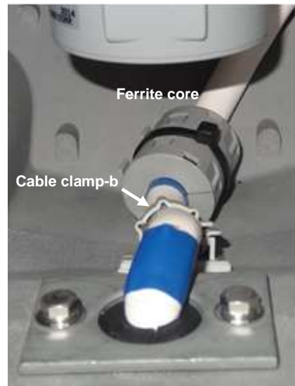
14) Clamp the cable by the cable clamp-b.
